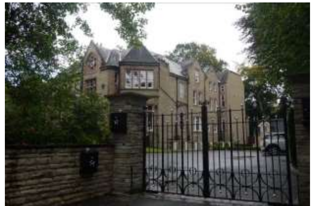
Large historic residential plots are harmed by inappropriately ornate modern railings, and excessive hard-standing
