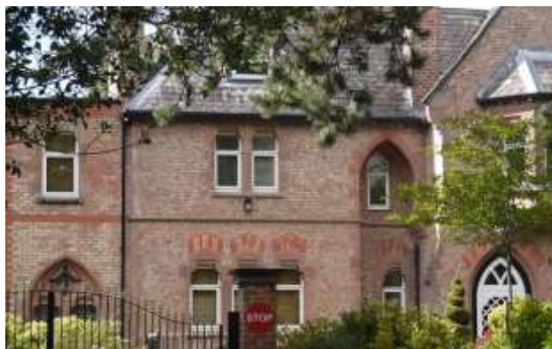
Gothic architecture with plate tracery and arched openings. Note the decorative slates and a high quality use of the local brown bricks.
