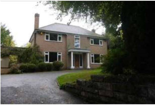
Late 20 th century development making use of simple classical details that do not fit in with the architecture of the Conservation Area at 6 Highgate Road
