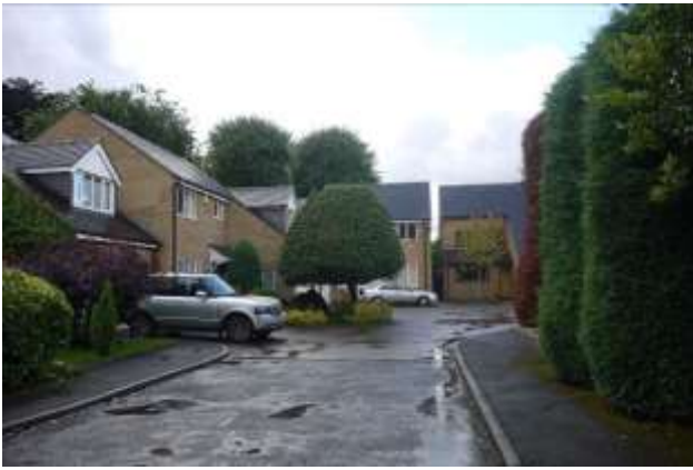
Devisdale Court, an example of a modern cul-de-sac development within Character Zone A, with high density development using modern materials and designs
