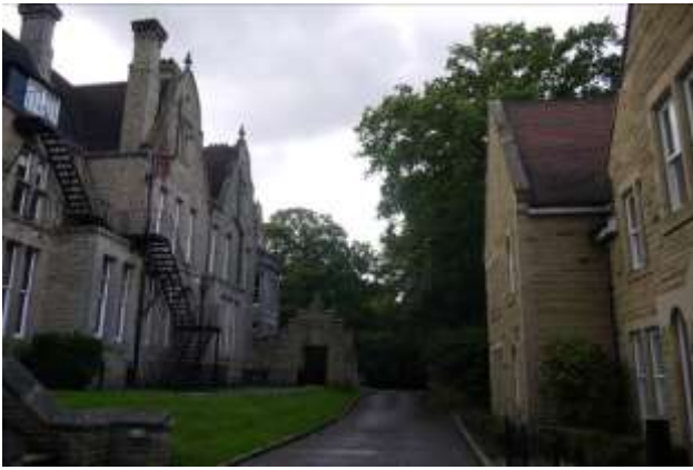
The historic Denzell House and more modern addition on the site, both making use of coursed, rough-faced stonework
