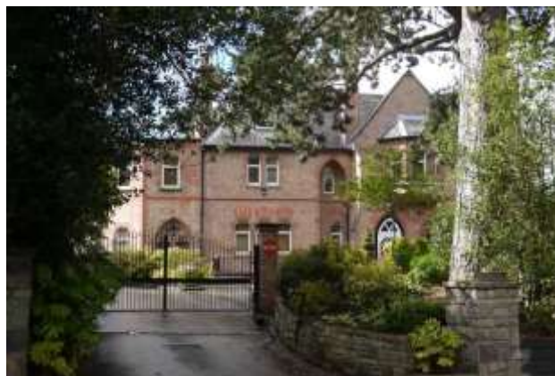
Typical materials include local brown brick, decorative Welsh slate, timber windows and stone details, Morningside, Highgate Road
