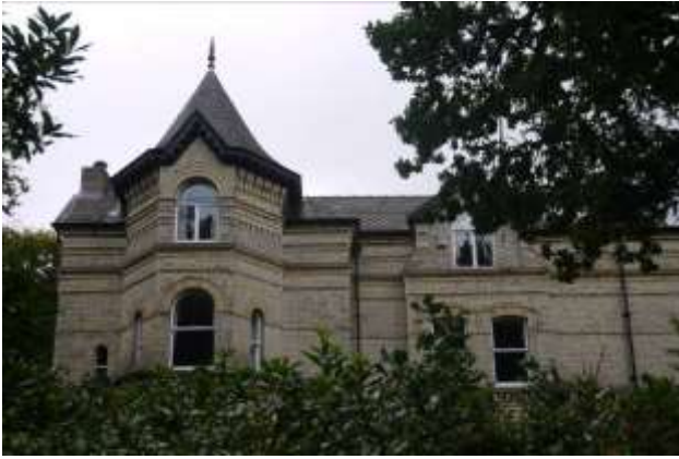
Turrets, dogtooth brickwork, rounded arches and decorative slate patterns are all local features of the area
