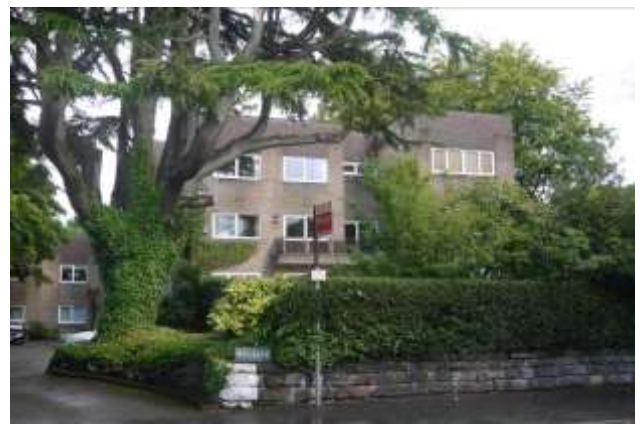
Westfield on St Margaret's Road is a modern development on an historic plot that is unsympathetic to its surroundings
